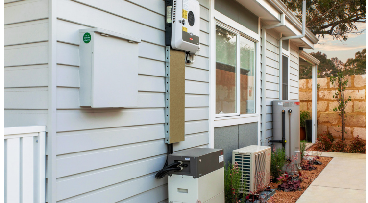
Battery and inverter connected to the Resort's embedded power microgrid
