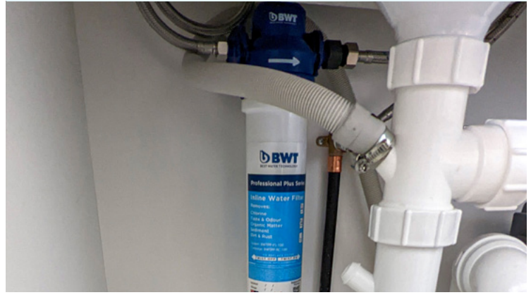
WFA HiFlow inline water filter system
