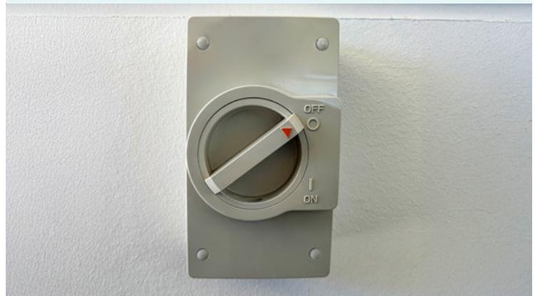
20-amp isolation switch to all carports/ garages suitable for electric vehicle charging
